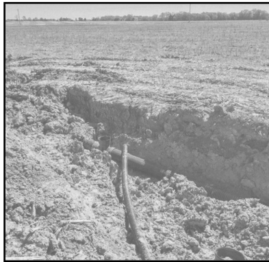
A drain tile partly uncovered.
